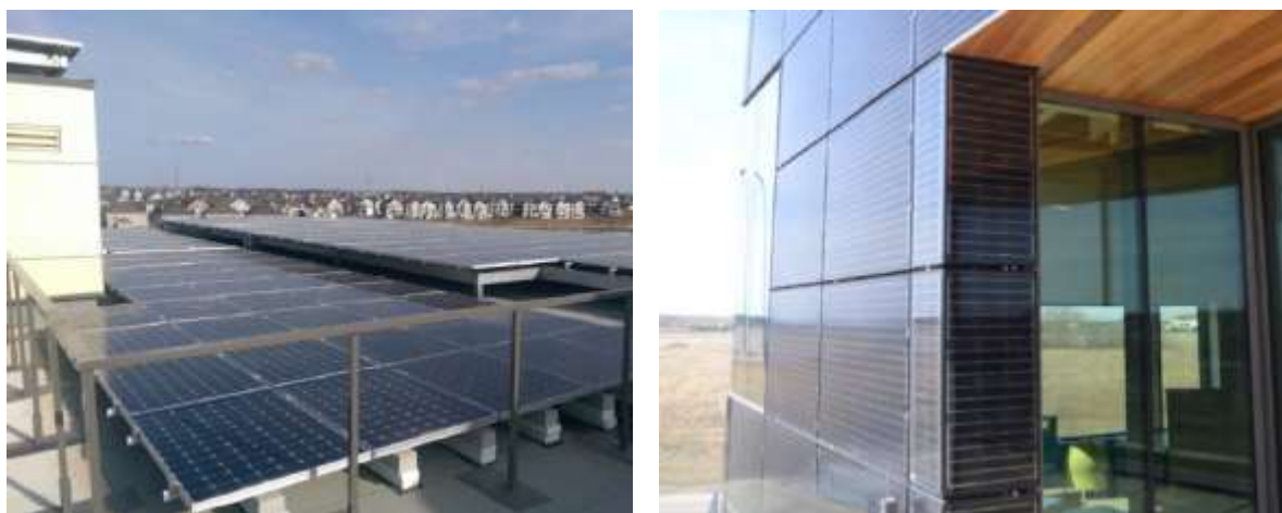
Fig 39: PV Panels on the Roof and Facade of the building (Manasc Issac Architects,2013)
