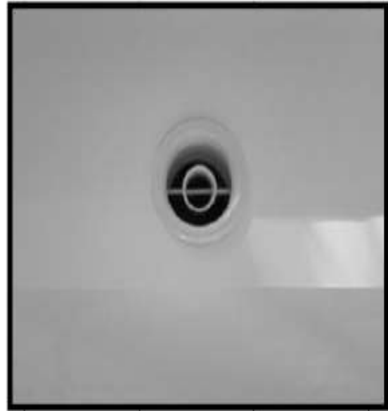
Fig 17: Current Fan Coil Unit (FCU)
