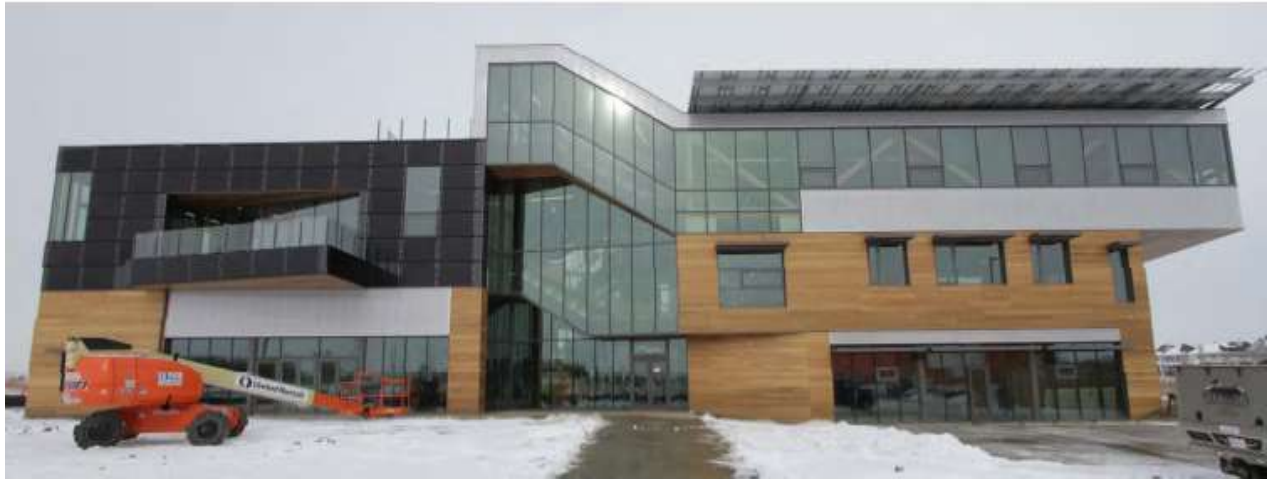
Fig 38: Facade (Manasc Issac Architects,2013)
