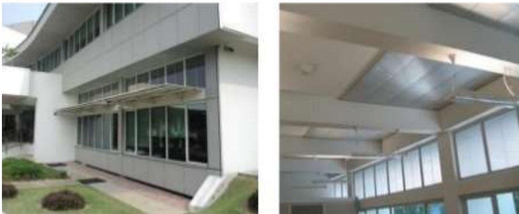
Fig 11: Exterior Overhangs and internal reflector ( http://www.slideshare.net/yassyed31/building-science-1-ptm-geo-2 )
