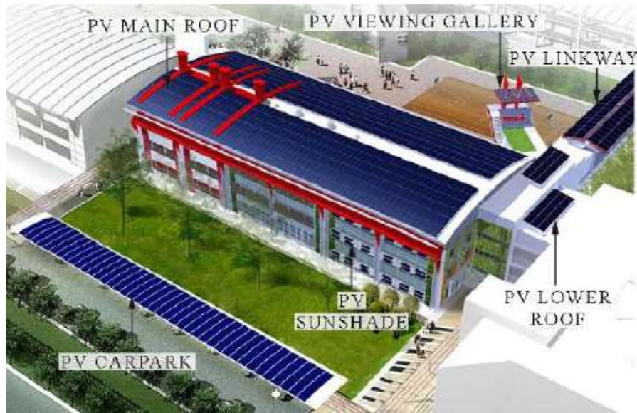
Fig 30: Integrated Photovoltaic (The Design, Development and Performance of a Retrofitted Net Zero Energy Building in Singapore, 2015)
