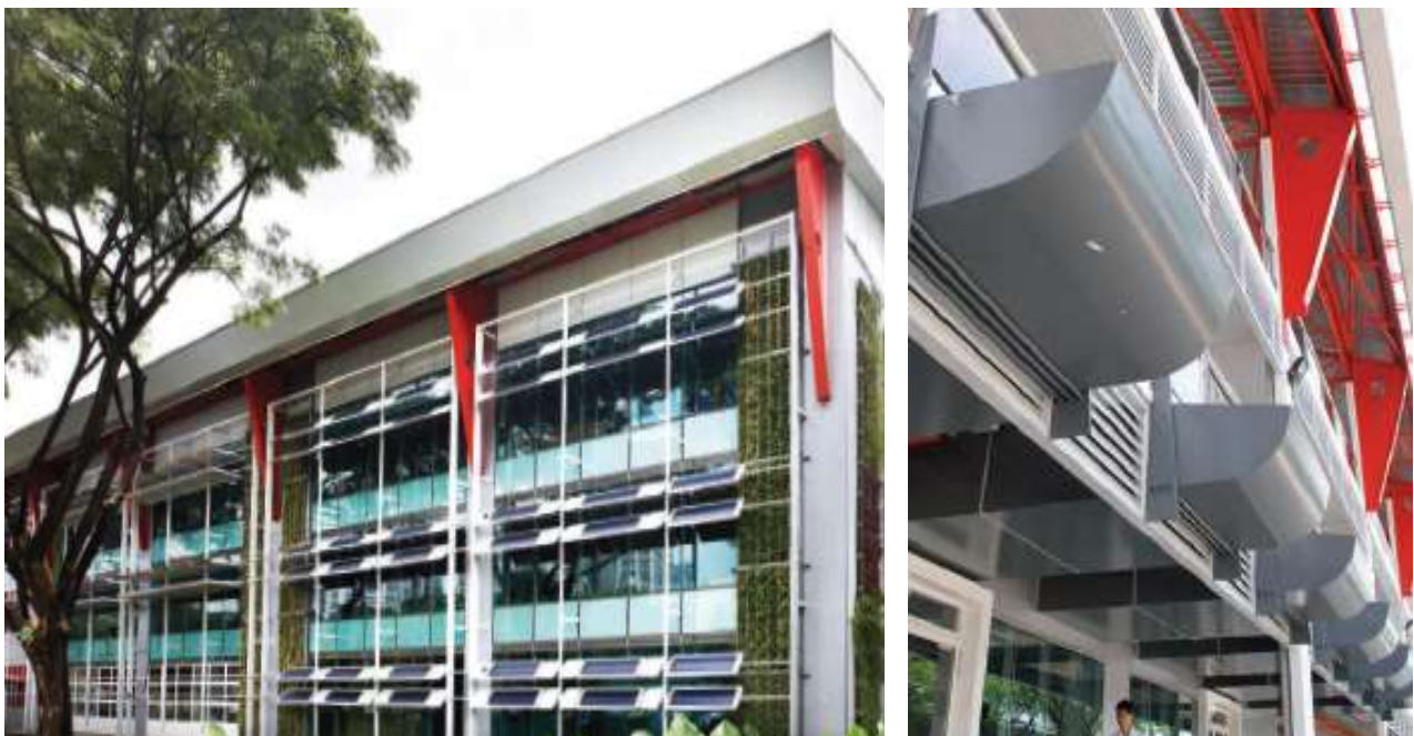
Fig 31: Façade Designed with passive strategies and Light Ducts (Building and Construction authority of Singapore, 2014)
