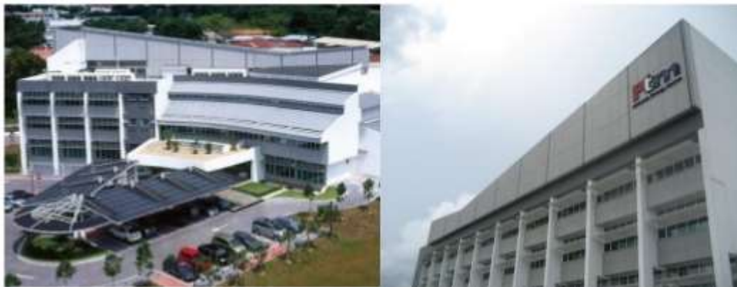
Fig 6: North and South facades http://www.greenbuildingindex.org/why-green-buildings.html )
